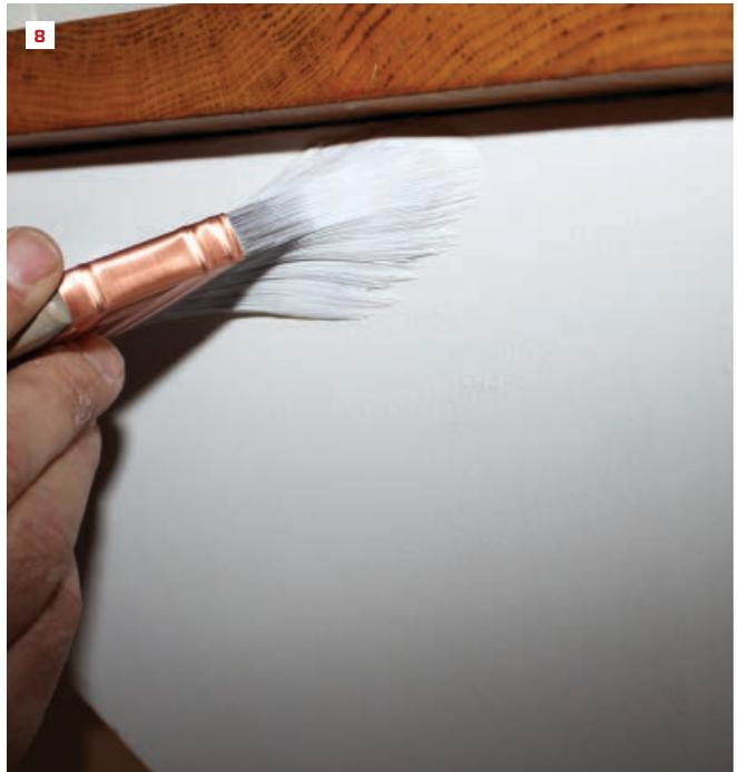
will pull a wider stroke, but the 2-inch will move more material. Brushing is a game of laying out material efficiently and getting it level in the fewest number of moves possible.
